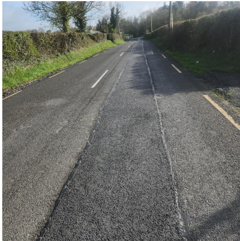
Plate 2-1: Castlecomer road completion works
